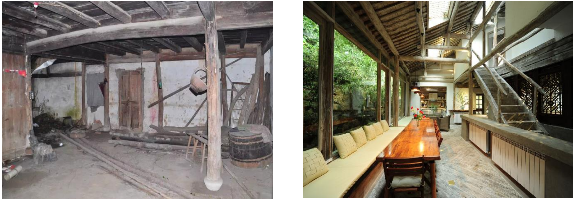
Fig.4-5. Modernization of the Traditional Residence Which Was Built in 1920 on Mogan Mountain, Deqing County, Zhejiang Province
