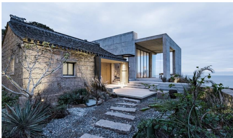
Fig.8. The Juxtaposition of Traditional Relics and Modern Structure in Dahuanglong Island, Zhejiang Province
